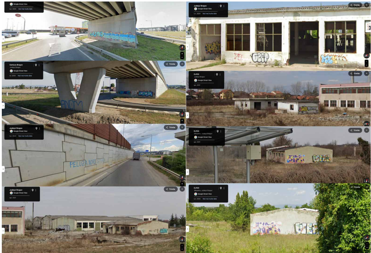
Figure 8: Braşov peripheral zones - bridges, abandoned buildings.
